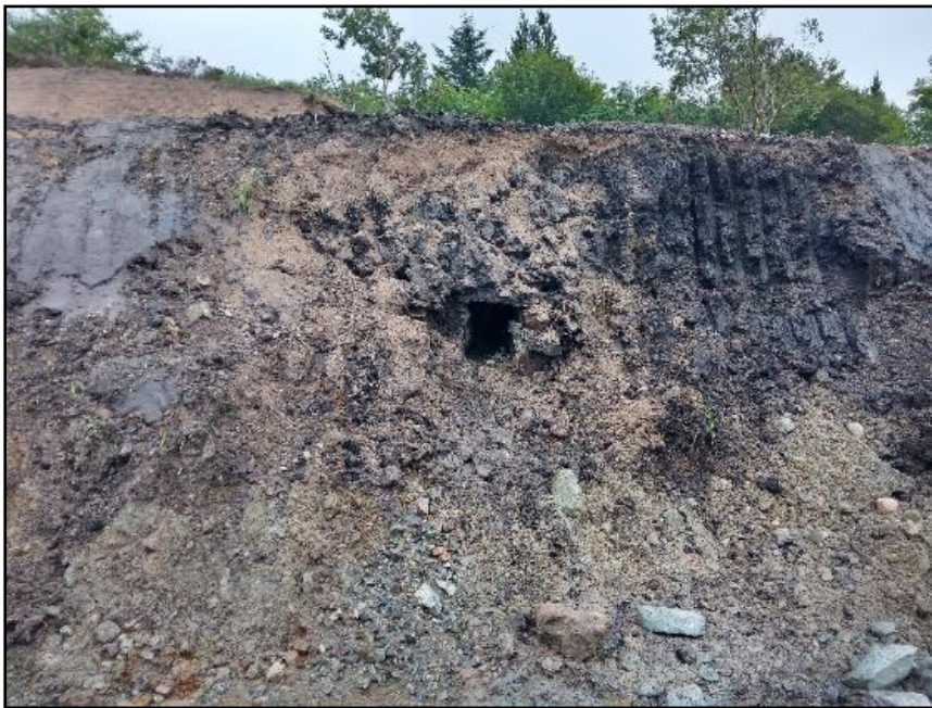
Plate 4 Exposed culvert in section face to north of site entrance
