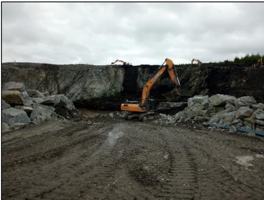
Plate 37 Borrow pit 1 in use as peat disposal area
