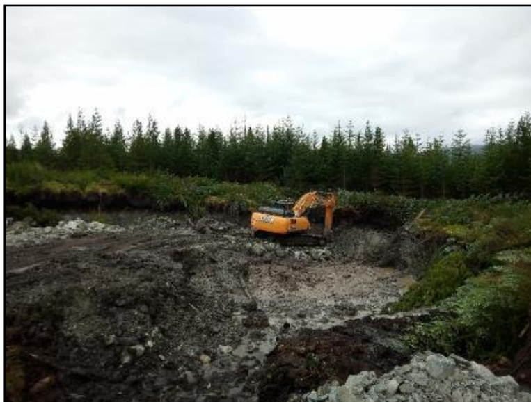
Plate 18 Looking north at excavation of turbine base at T8
