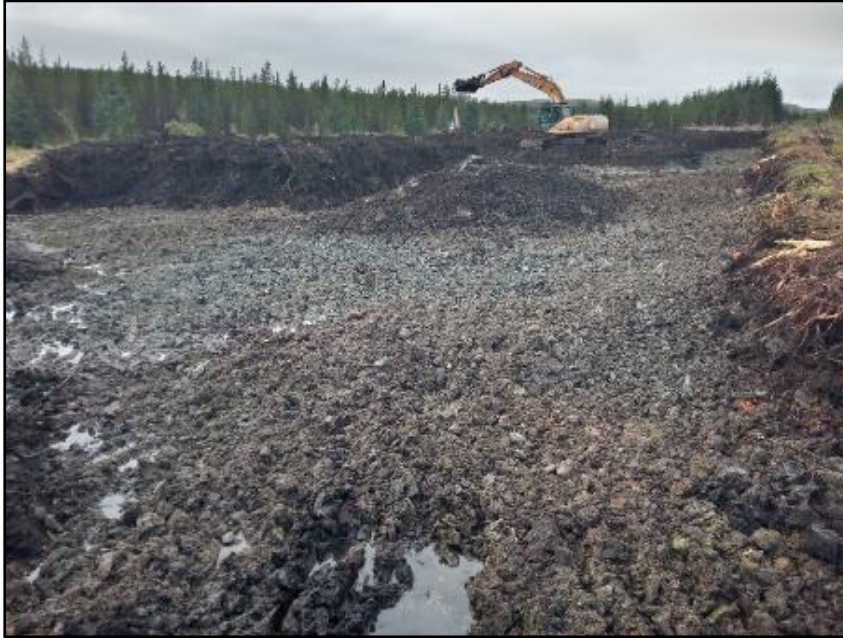
Plate 33 Looking southwest at T18 hardstand excavation
