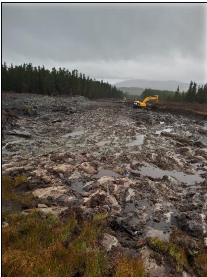
Plate 35 Looking west across T19 hardstand post topsoil stripping
