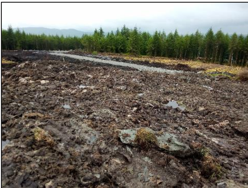
Plate 16 Looking northwest at T6 following base and hardstand strip
