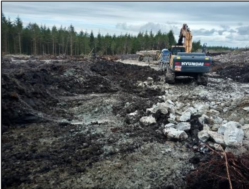
Plate 15 Looking west during excavations at T6
