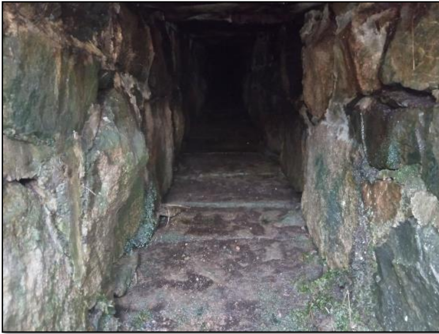
Plate 5 Interior of culvert showing flagstone flooring and mortared wall
