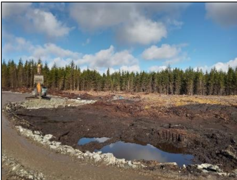
Plate 10 Looking northwest at excavation of turbine base at T2
