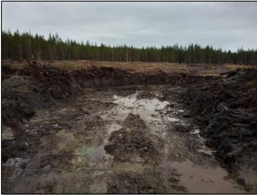
Plate 9 Looking east at excavations of hardstand at T2
