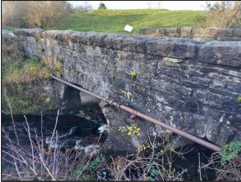
Plate 51 Looking west at road bridge NIAH Ref. 40909424
