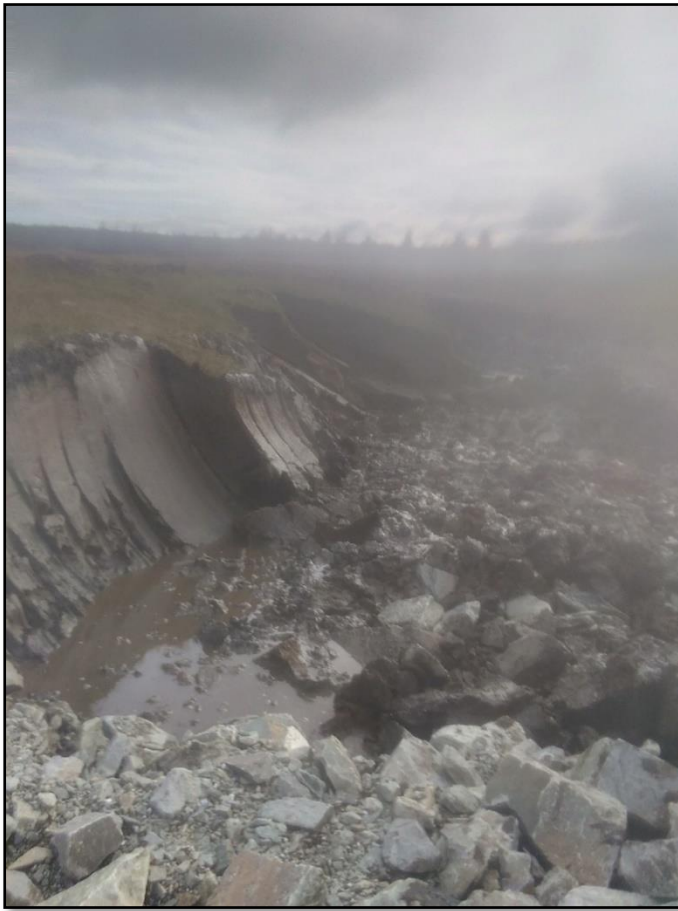
Plate 55 Peat section face in T16 hardstand extension
