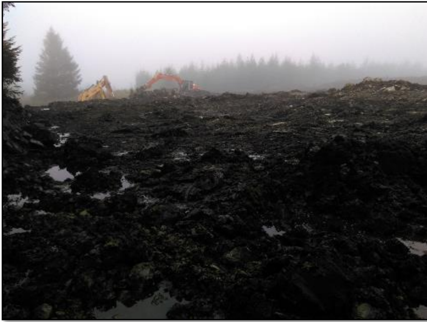
Plate 42 Peat Storage Area located southeast of the substation
