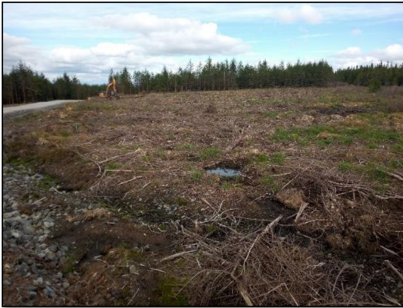
Plate 13 Looking northeast at site of T5 pre peat excavation
