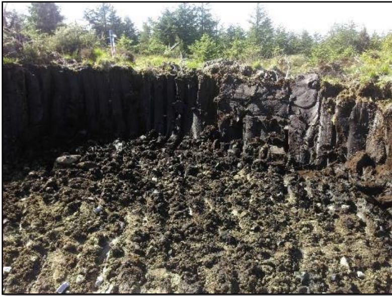
Plate 26 Southeast-facing peat section at hardstand for T12
