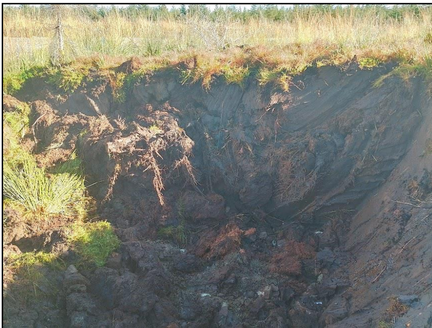
Plate 57 Looking west at peat section in new road to T9
