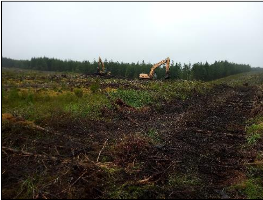
Plate 19 Looking west at site of T9 pre-excitation
