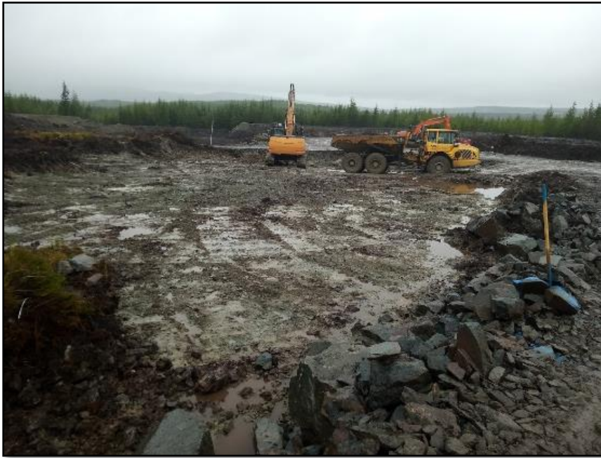
Plate 29 Looking northwest at T15 hardstand
