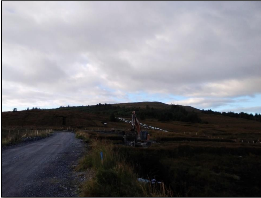
Plate 56 Looking east at Site Access Road Realignment
