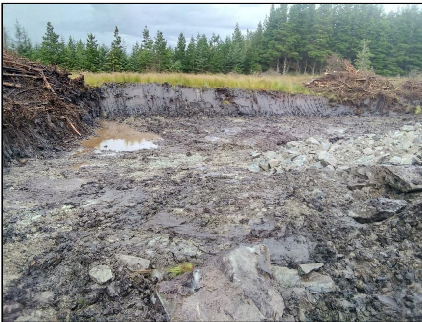
Plate 54 Looking west at Borrow Pit post peat excavations
