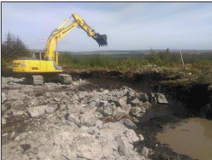
Plate 25 Looking north at peat excavations for turbine base at T12
